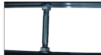
Fig 2. Connection of upper to lower profile by means of stud bolts which are fastened with a self locking nut.
